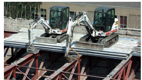
JOCK HARTY ARENA, QUEEN'S UNIVERSITY DEMOLITION & ASBESTOS ABATEMENT, KINGSTON, ONTARIO
