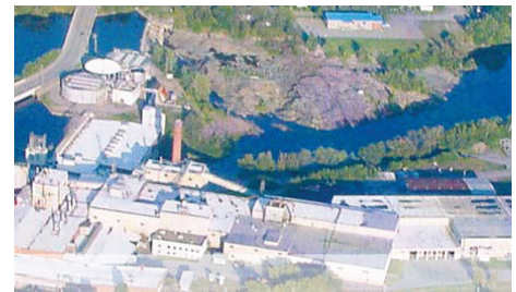
WEYERHAUSER PULP & PAPER MILL DEMOLITION, ASBESTOS REMOVAL AND SOIL REMEDIATION STURGEON FALLS, ONTARIO
